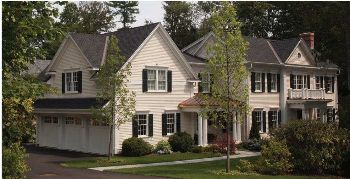
Classic Raised Panel, 2-section with center midrail, 4" Lag Pintels with 6" L-hinges, Acorn bullet catches & Rat tail holdbacks
